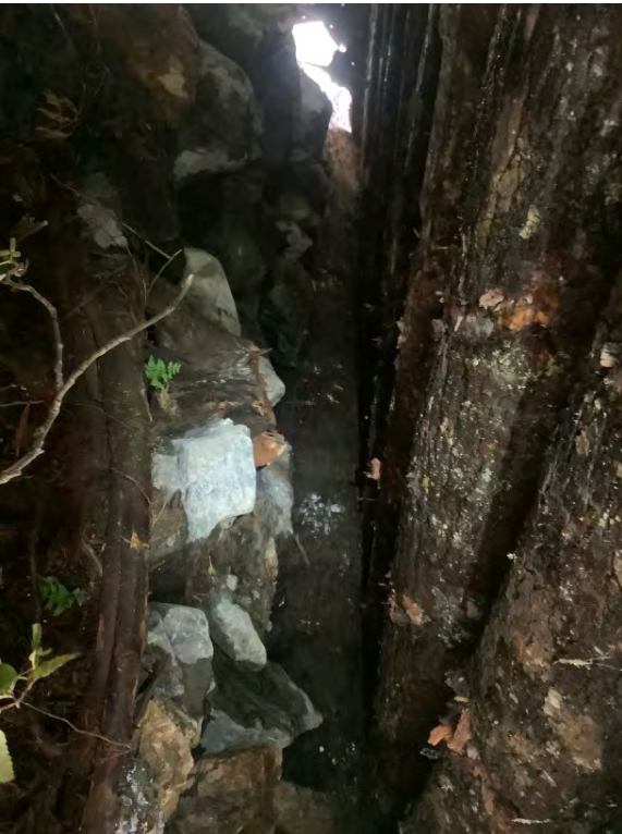
Right Bank Abutment when facing downstream
